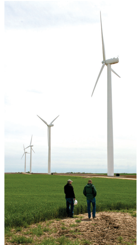
The Department of Agriculture provides grants to farmers and ranchers for renewable energy development. Photo from Native Energy, Inc., NREL 17589
