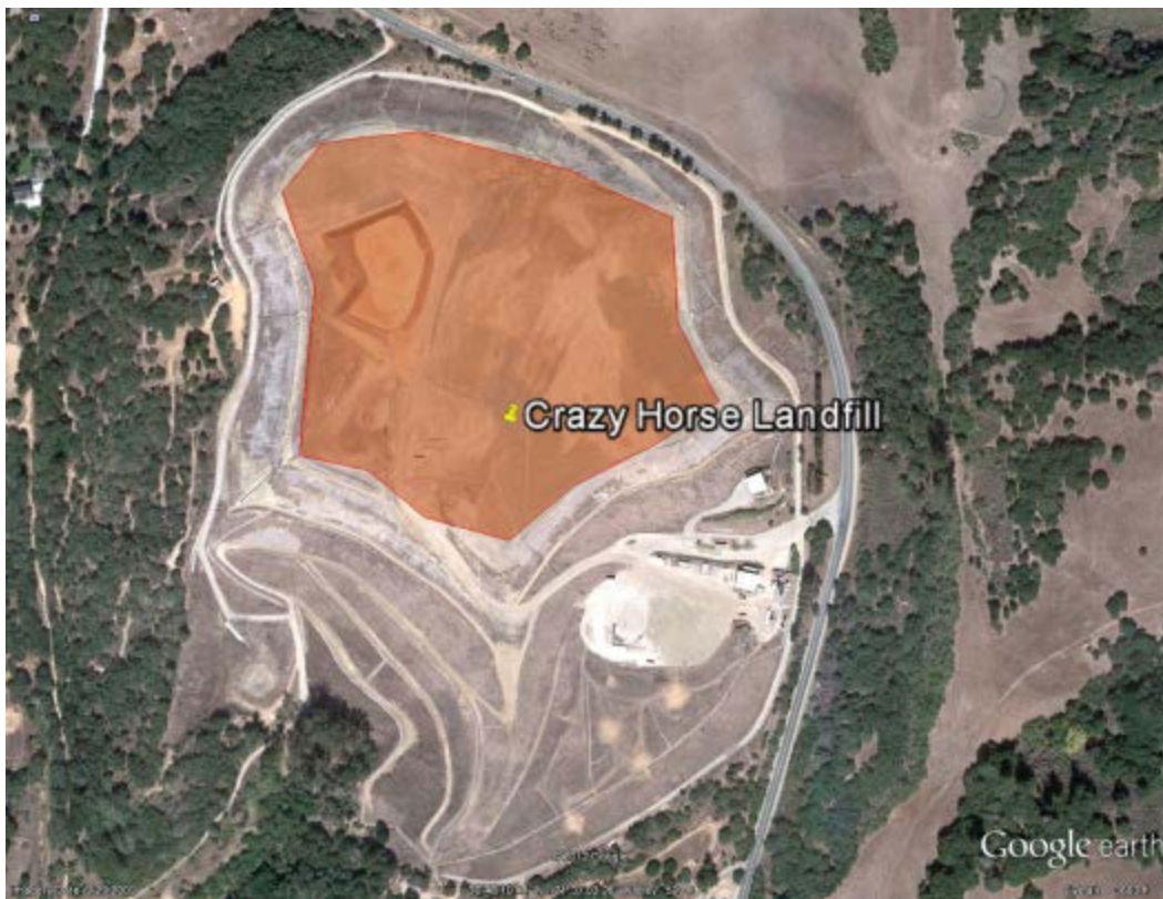
Figure 7. Aerial view of the feasible area (orange) for PV at the Crazy Horse Landfill site
