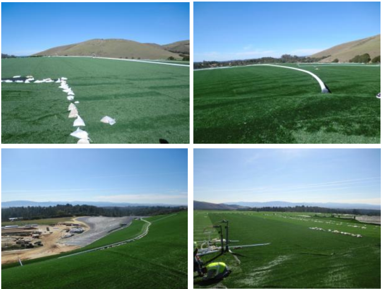
Figure 6. Views of the feasible area for PV at the Crazy Horse Landfill. Photos by Blaise Stoltenberg, NREL
