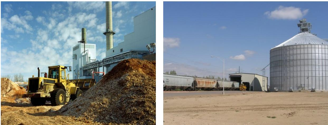
**Figure 3. Biomass storage options: fuel yard and fuel silo. Photos by (left) Warren Gretz, NREL 04376 and (right) Gerry Harrow, NREL 15041**
