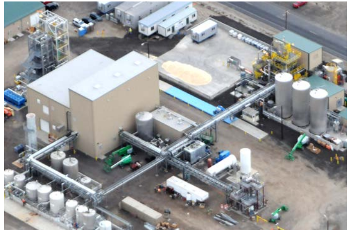
ZeaChem’s 250,000-gallon-per-year cellulosic biorefinery in Boardman, Oregon, will deploy its hybrid biochemical and thermochemical technology to produce fuel-grade ethanol from poplar and other feedstocks. Photo from ZeaChem
