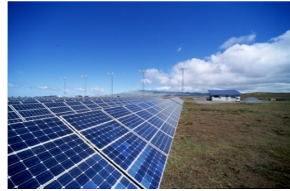
Source: NREL PIX-13823
