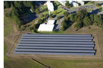
Source: NREL PIX 17395
