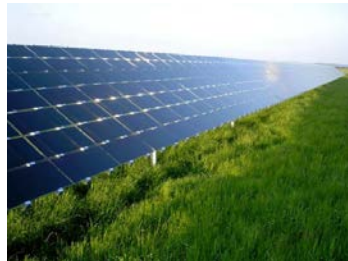
Source: NREL PIX 14726
