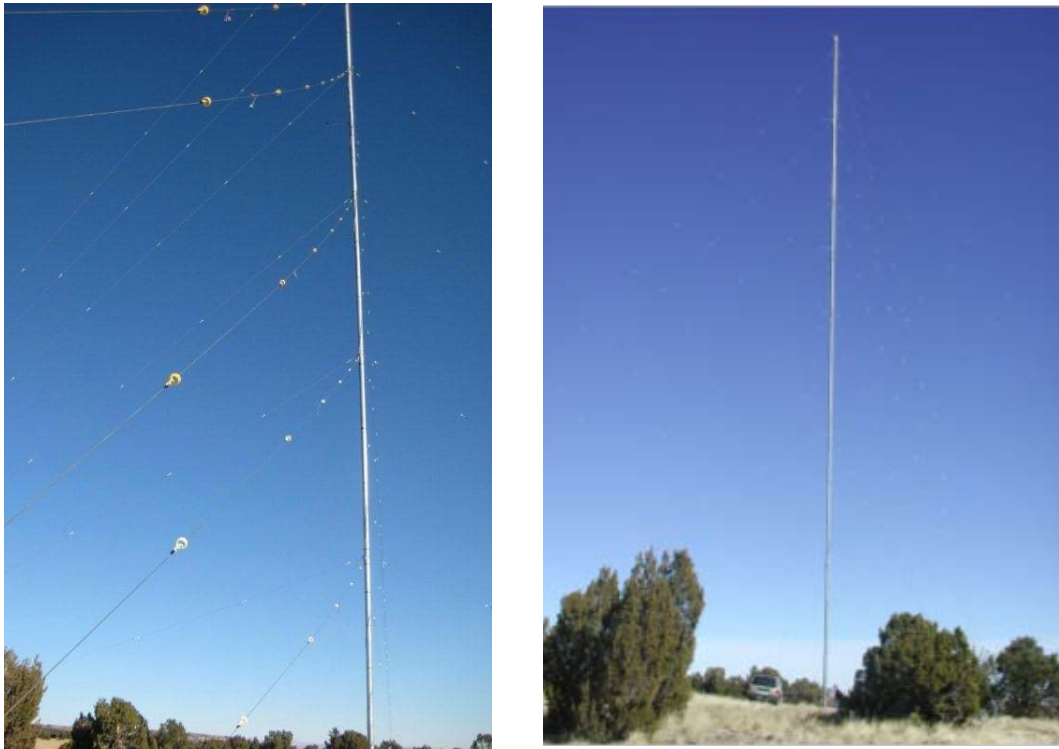
Figure 23 Fort Carson 50m met tower with bird diverters. Photo credit: Robi Robichaud, NREL
