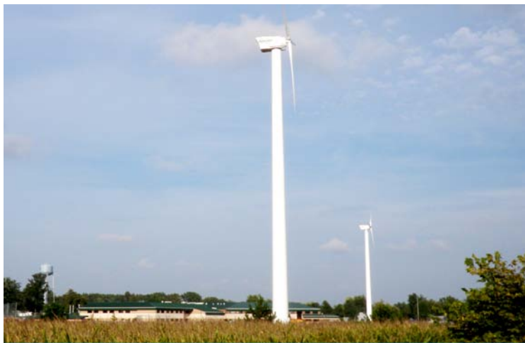
Two 100-kilowatt Northern Power Systems wind turbines provide on-site energy generation for the Upper Scioto Valley School in McGuffey, Ohio. Photo courtesy of NexGen Energy Partners, LLC, NREL/PIX 16741
