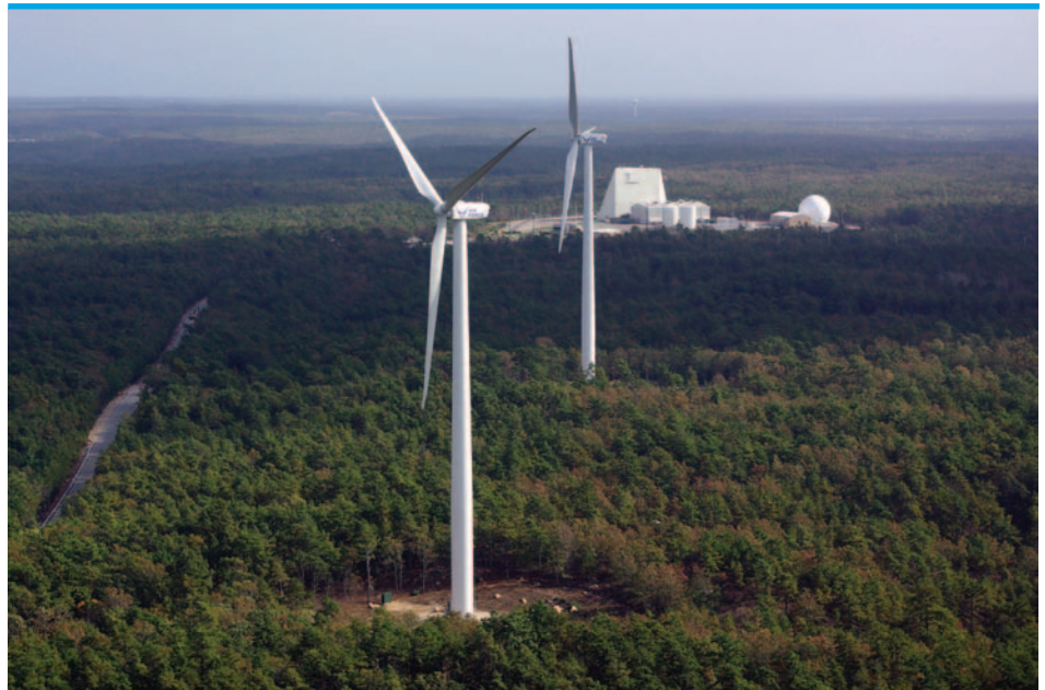
Two 1.5 MW net-metered wind turbines provide power for the clean-up project at MMR. Photo from Air Force Center for Engineering and the Environment
