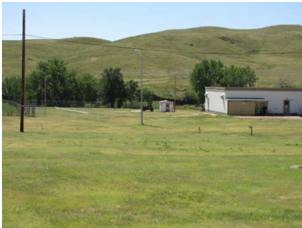
Waste Water Unit
