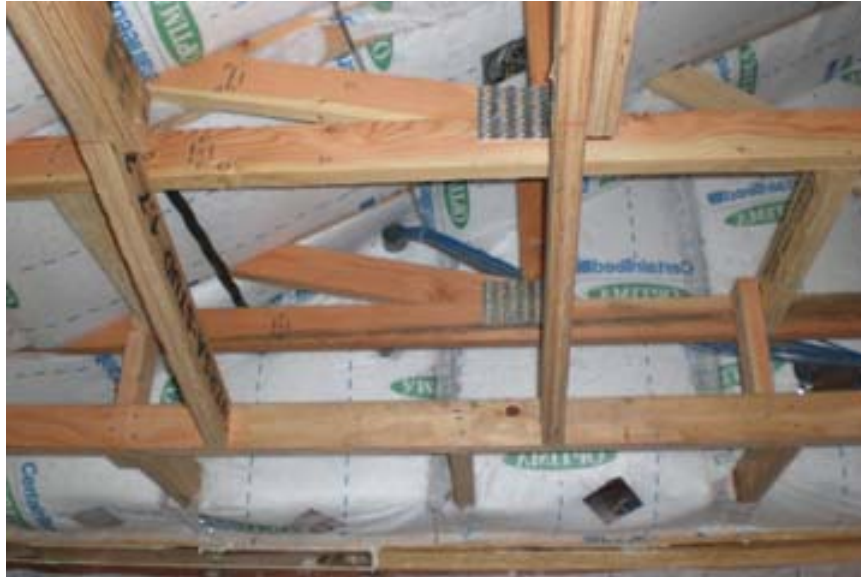
Figure 6: Netted blown insulation at roof and kneewall
