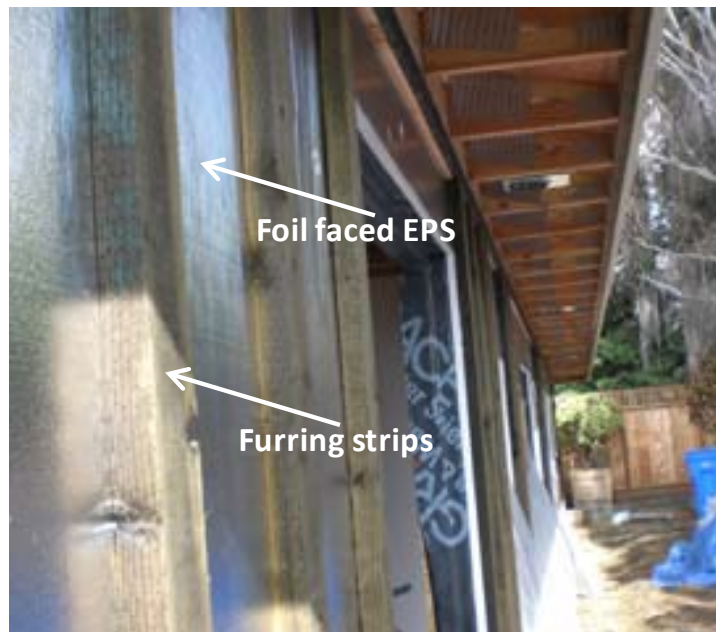
Figure 5. Exterior wall showing foil-faced EPS and furring for siding
