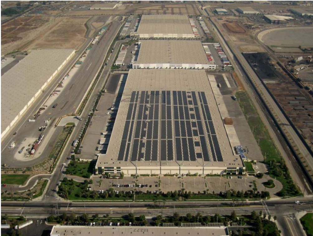
Figure 5-10: View of the 2.0 MW PV System Installed on a Warehouse Rooftop in Fontana, California (Photo courtesy Southern California Edison)
