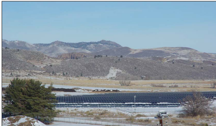
Figure 3-2: PV System at Colorado State University Foothills Campus
