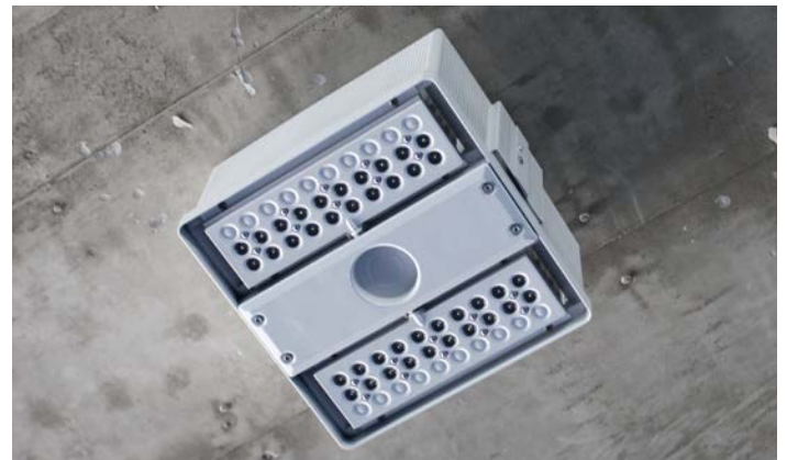
71-Watt LED fixture used in the NREL parking structure.
