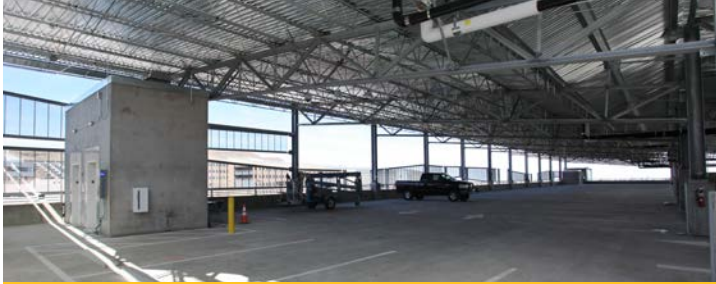
Perspective showing the PV roof structure on the top floor and perforated metal panels for an open façade with some weather protection.
