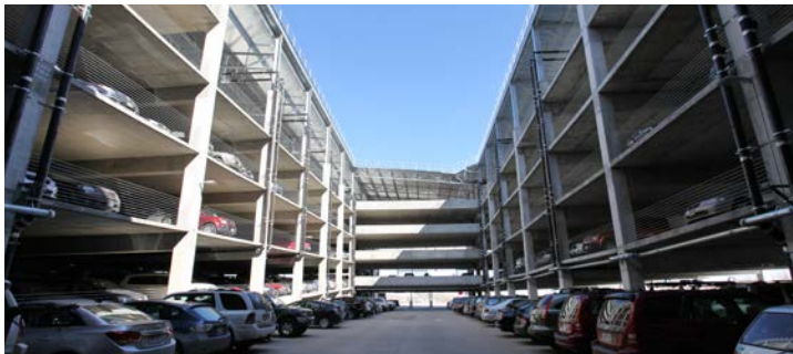
Light well perspective showing light-colored concrete and cable barriers for increased daylight saturation inside the structure.
