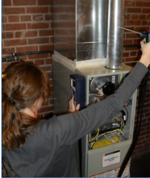
Figure 4. Draft pressure testing using combustion analyzer
