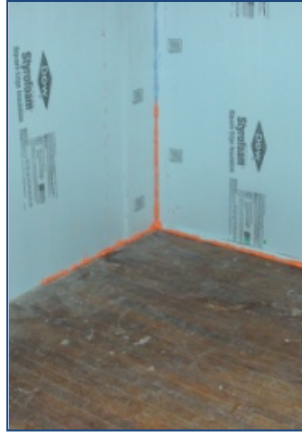
2. Install rigid foam and air seal.
