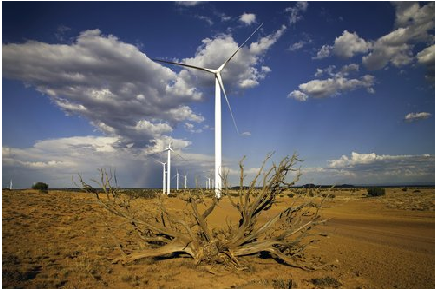
Photo from Iberdrola Renewables, NREL PIX 16072
