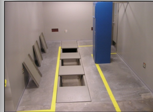
Utility trench from corridor into PDIL
