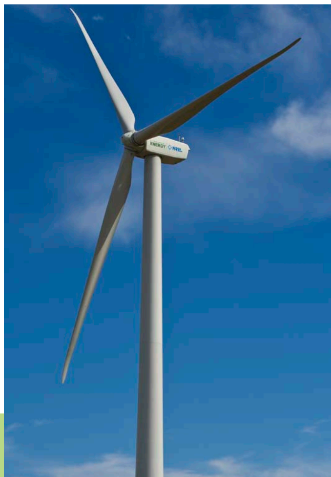
Photo by Dennis Schroeder, NREL/PIX 20373
