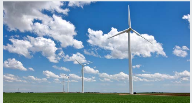
Winds that destroyed Greensburg are now supplying power to the city, thanks to the 12.5-megawatt Greensburg Wind Farm, which was erected in early 2010. Photo from Native Energy, Inc., NREL/PIX 17592
