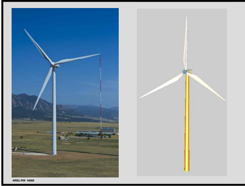
Figure 1. (left) ALSTOM ECO-100 turbine at NWTC. (right) turbine simulation in S4WT.
