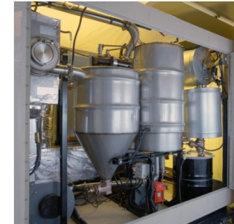
Photo by Kim Yost, NREL/PIX 11915
