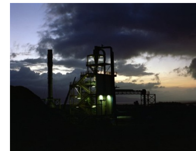
Photo by Warren Gretz, NREL/PIX 03793
