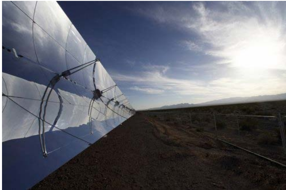
Photo by Geri Kodey, NREL/PIX 14383
