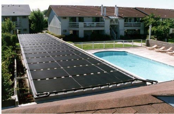
Photo from Gen-Con, Inc., NREL/PIX 09320
