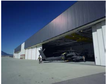
Photo by Warren Gretz, NREL/PIX 00595
