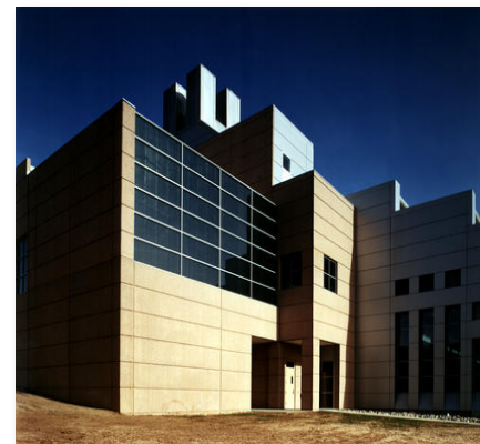
Trombe Wall, NREL. Photo by Warren Gretz, NREL/PIX 01693,
