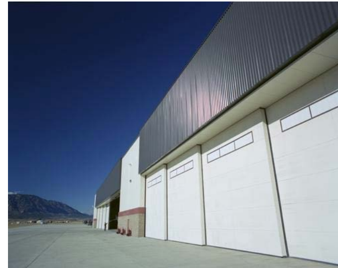
Photo by Warren Gretz, NREL/PIX 14383
