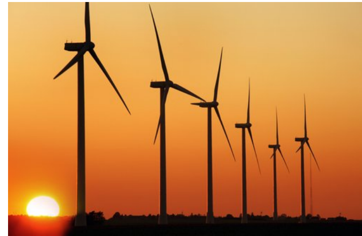
Photo from Alstom 2010, NREL/PIX 18207
