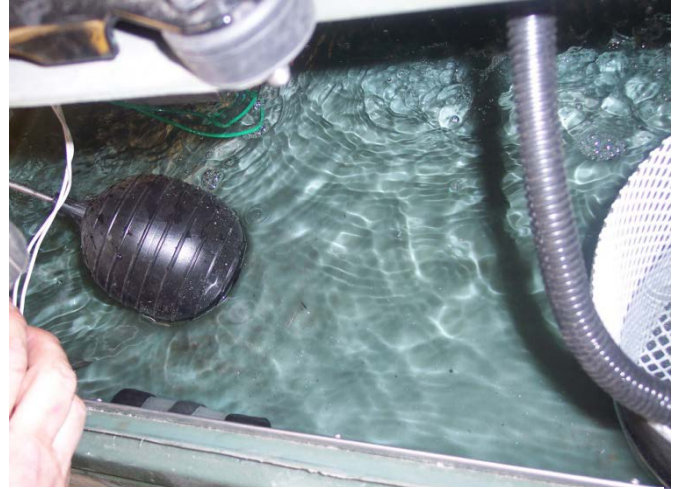
Figure 8: Float to adjust water sump level
