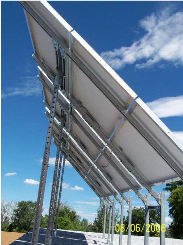
Fig. 4. Photograph of the back row of panels on the detached garage showing the 40° tilt.
