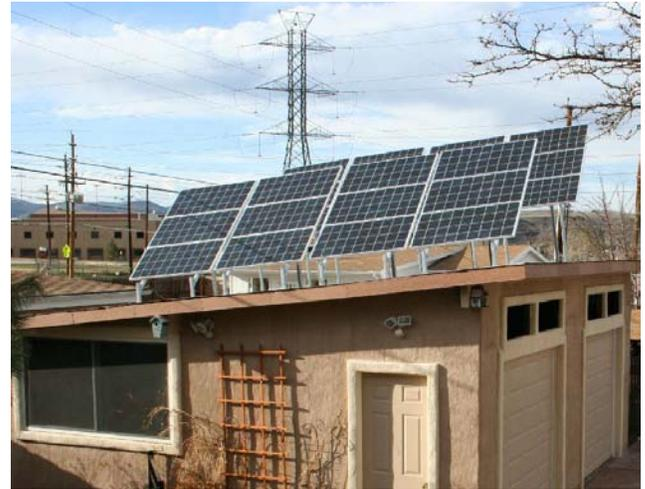
Fig. 5. Photograph shows shadows of power lines that are cast across the panels in the late afternoon.
