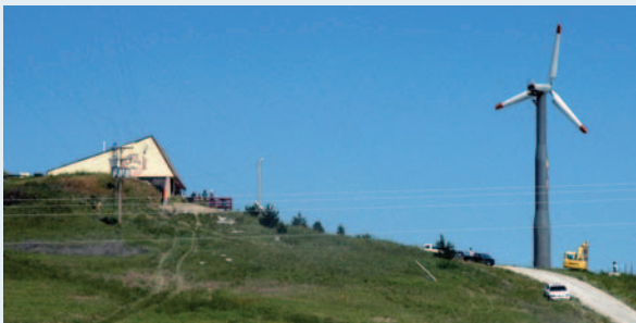
Workers attach the blades of a refurbished wind turbine that powers the KILI radio station at the Pine Ridge Reservation in South Dakota. Photo by Bob Gough, NREL/PIX 15954
