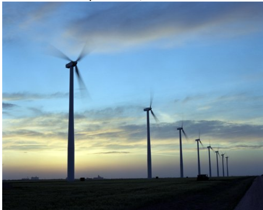
Photo by Warren Gretz, NREL/PIX 11188
