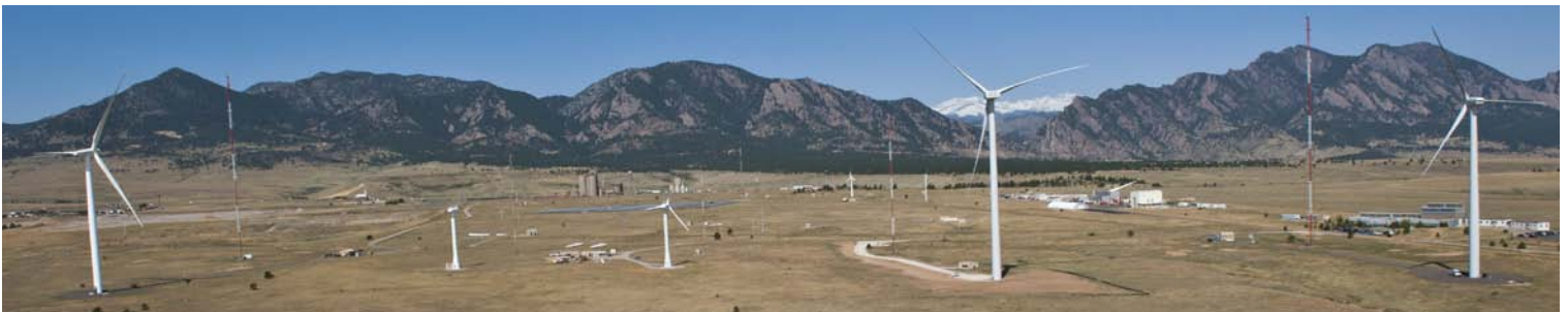
Aerial photo of the NWTC, located at the base of the Rocky Mountains in Colorado. Photo by Dennis Schroeder, NREL/PIX 19065
