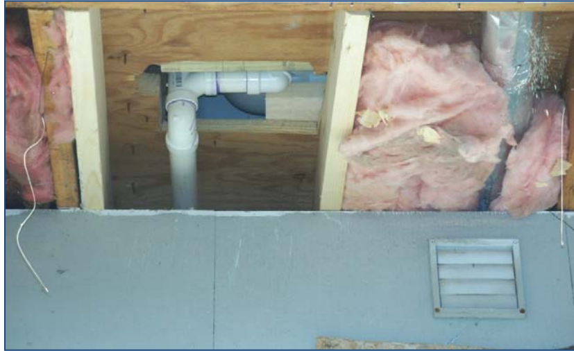
Figure 4. Existing conditions of cantilever floor area per visual inspection
