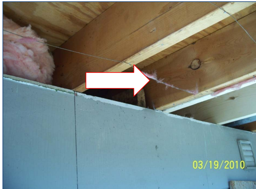
Figure 9. Cantilevered floor blocking training sheet
