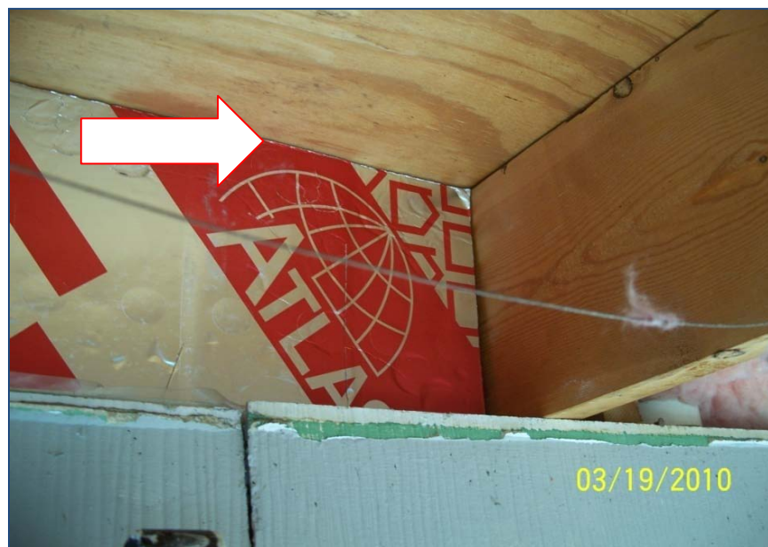
Figure 10. Cantilevered floor air sealing training sheet
