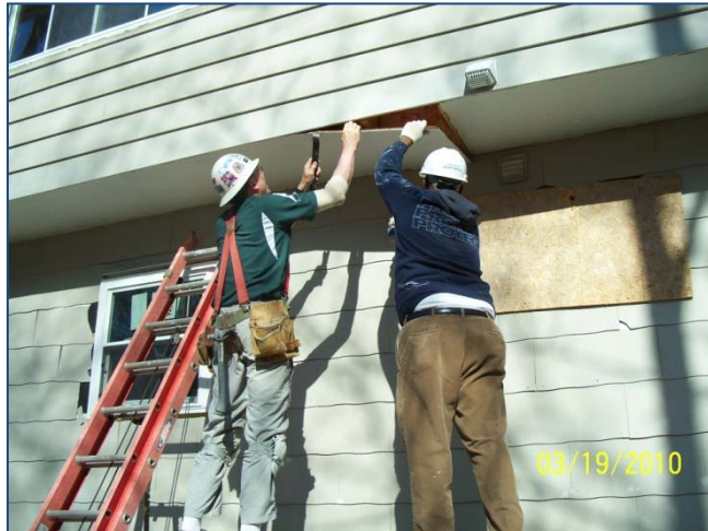
Figure 8. Cantilevered floor blocking, air sealing, and insulation
