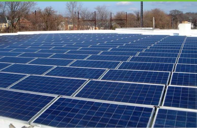
The Bushnell Company in the Germantown neighborhood of Philadelphia uses an 85-kW rooftop PV installation. Photo from Mercury Solar Solutions, NREL/PIX 18064
