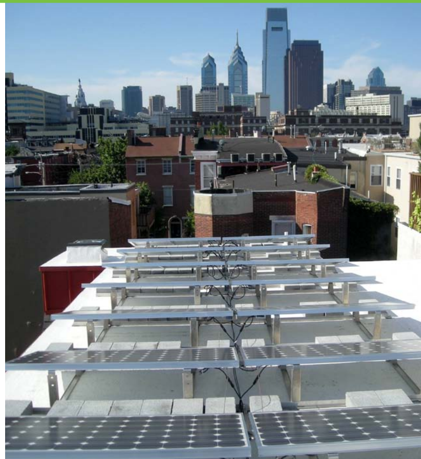
The Philadelphia skyline is a beautiful backdrop to a 3-kW PV rooftop installation in the Center City District. Photo from Mercury Solar Solutions, NREL/PIX 18063
