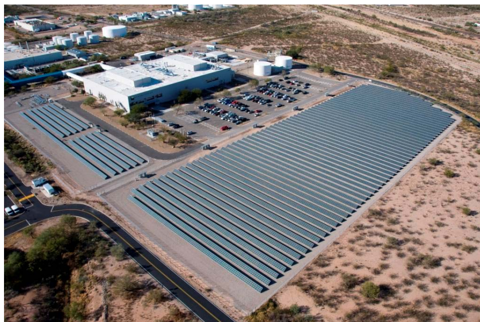
Fig. s3. The GSE factory in Tucson, showing the ground-mounted 750 kWp CIGS power field in AZ. (Credit: Global Solar Energy)
