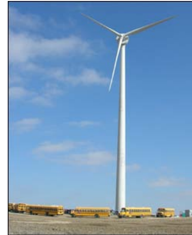
Dedication of a 900-kW Americas Wind Energy wind turbine installed in Wray, Colorado by the Wray School District RD-2. Photo by Ian Baring-Gould, NREL/PIX15461
