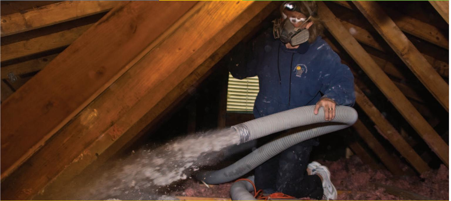
A weatherization crew member blows dense pack insulation into the attic and wall cavities of a client's home.
