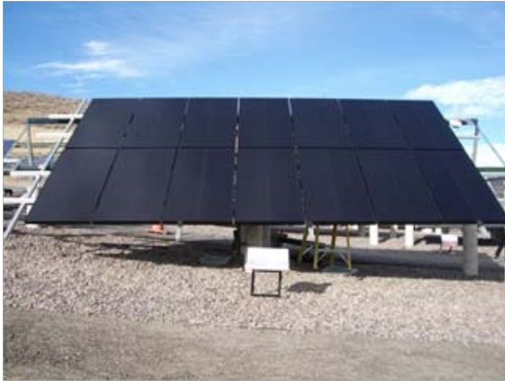
Shell Solar E80-C modules deployed at NREL. Photo credit: Harin Ullal, NREL PIX 14725
