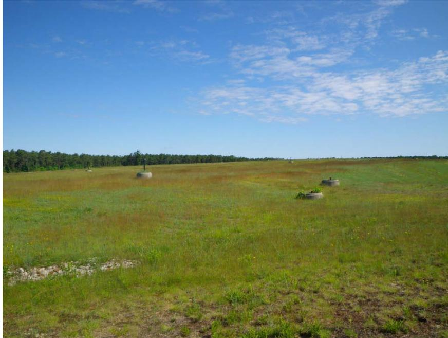
**Figure 7. Landfill cap with relatively shallow slope**
