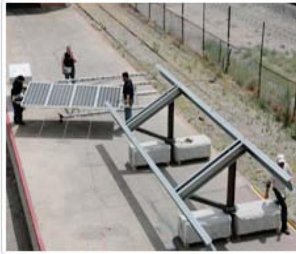
**Figure 9. A ballast-weighted system using two precast concrete weights**
