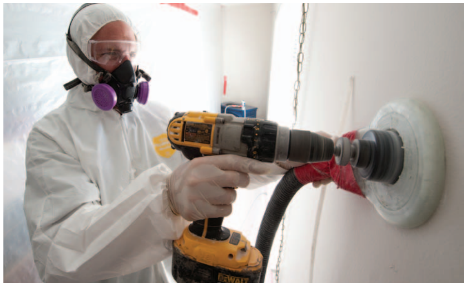
A weatherization worker uses safety equipment that captures all dust in a home contaminated by lead paint. Healthy homes experts contributed to the Workforce Guidelines for Home Energy Upgrades to address occupant and worker safety issues. Photo from NREL/PIX 17966
