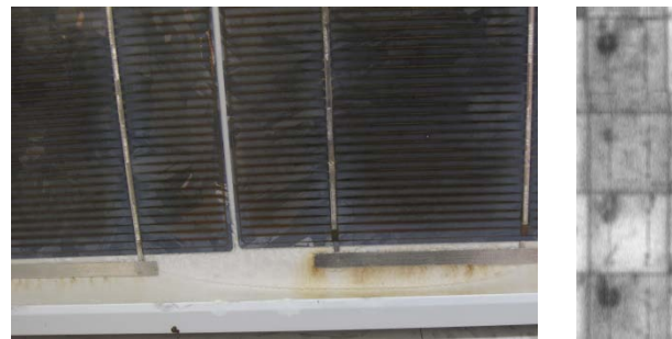
Figure 3. Left, image of a module after 2000 hrs. in damp heat with + 600 V applied to the active layer with respect to the grounded module frame. There is evidence of grid finger and aluminum frame corrosion, metal ionic transport from the bus strap, and occasional delamination. Right, electroluminescence image of a four-cell region of this module, indicating darkening and degradation at positions around the rear bondpads.
