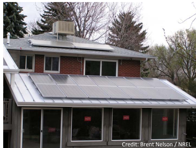
'Typical residential installation'. 2x7 mSi panels
