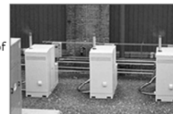
Hydrogen PEM fuel cells are leading candidates for use in fuel cell vehicles. Today's commercially available PEM fuel cells are particularly appropriate for low-power applications requiring intermittent backup.
