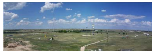
West Texas A&M University small wind turbine test field. PIX# 17242.
