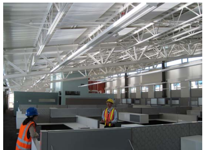
Figure 7 Example of the RSF's daylit interior
