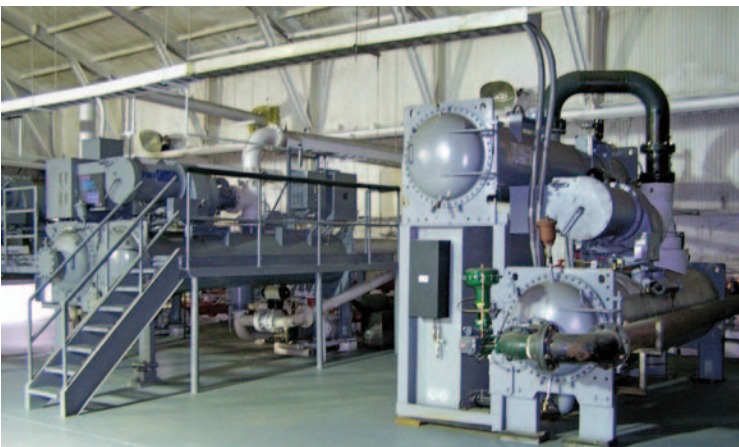
Chena Hot Springs Resort, in Alaska, uses the lowest temperature geothermal resource for commercial power production in the world by utilizing Organic Rankine Cycle units, shown here.
