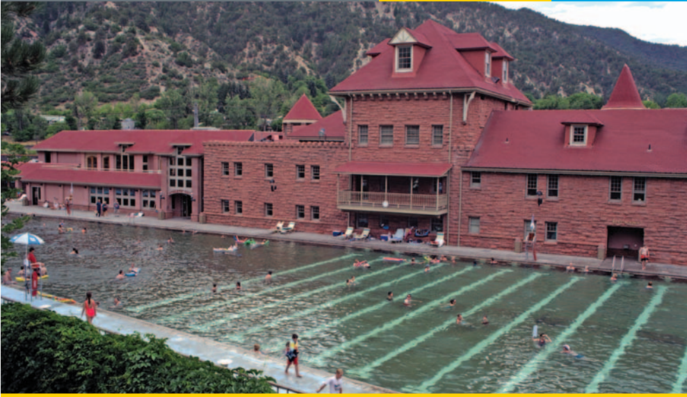
The 58,000-square-foot Hot Springs Lodge and Pool in Glenwood Springs, Colorado, uses a geothermal heat exchanger system with its hot surface spring to provide space heating, domestic hot water, and snow melting. PIX07931
