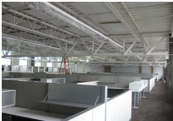
Figure 5: RSF Construction Photo
