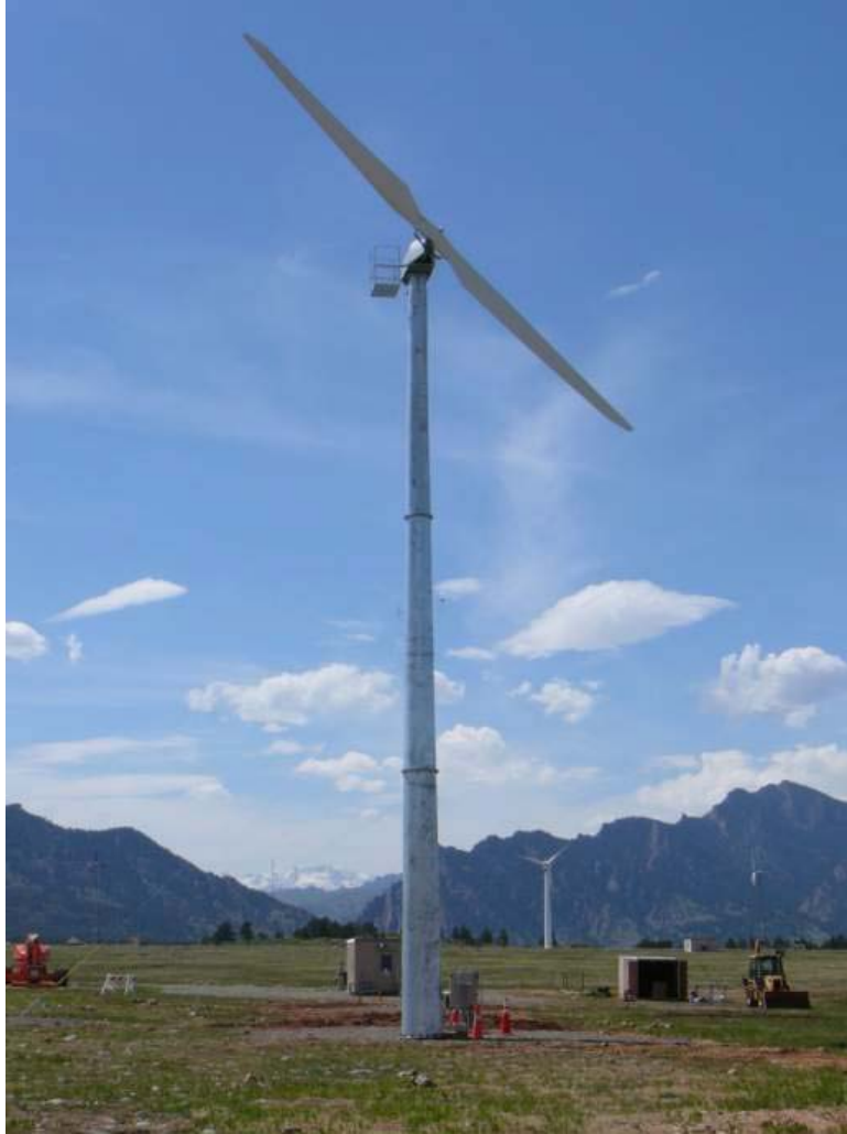
Figure 2. Gaia-Wind 11-kW test turbine at the NWTC
