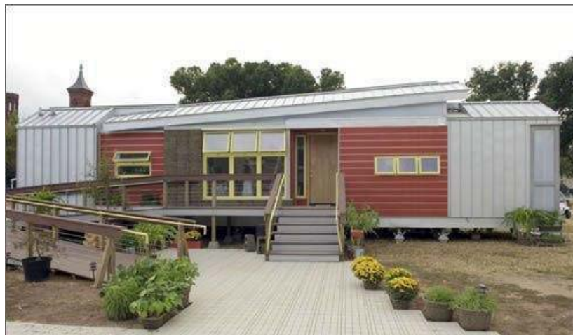
Figure 25. The Silo Eco-Home is built similarly to a grain silo, which was one of the few structures left standing in Greensburg after the tornado. On April 9, 2009, the builder (Armour Homes of Bushnell, Florida) tested the home's ability to withstand pressure by dropping a 1980 Honda Civic on the roof from a height of 60 ft. The home, unlike the car, was undamaged.
