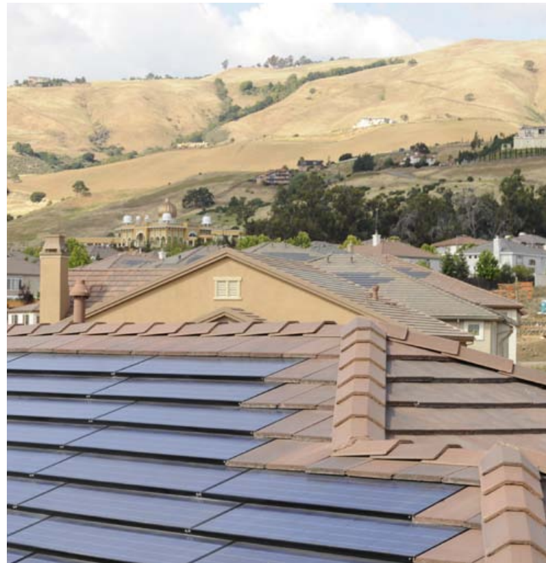
Energy Tile™, BP Solar's building-integrated product, is featured in homes by PinnBrothers in the Orchard Heights Community of San Jose, California. (Photo courtesy of PetersenDean)
