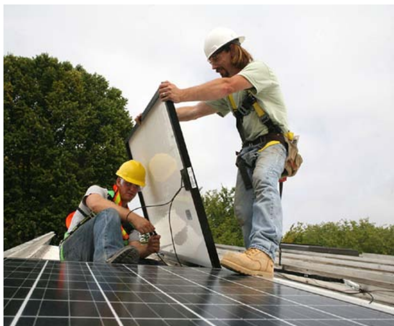
Harold Remlinger and Brian Eady install solar panels on the roof of the Solar Decathlon 2007 Lawrence Technological University house. (Credit: Kaye Evans-Lutterodt/Solar Decathlon)
