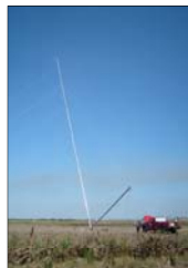
Installation of 50-m Met tower by AEI of West Texas A&M at GSA Border Station site in Donna, TX.
