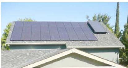
The back of the home features a 3.85 kilowatt rooftop photovoltaic system which, in conjunction with a solar thermal system and energy efficiency measures, helps reduce utility bills by 80%.
