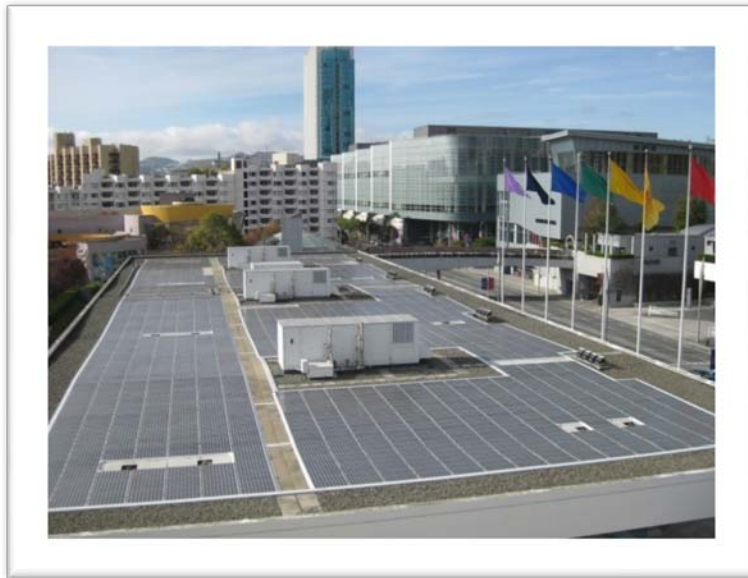
Figure 4. A Moscone Center Rooftop Loaded with PV Panels
