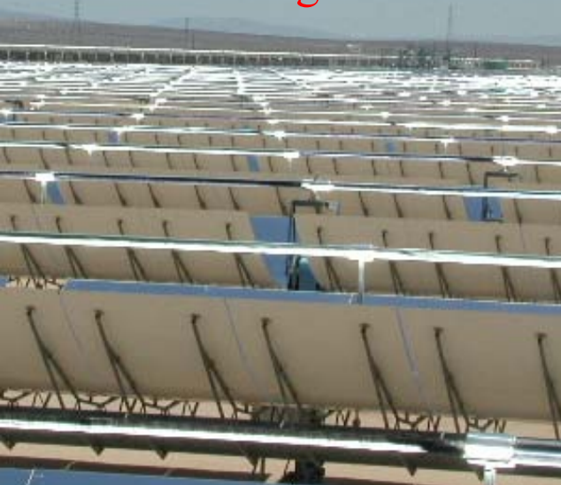
Compact Linear Fresnel Reflector (CLFR)
