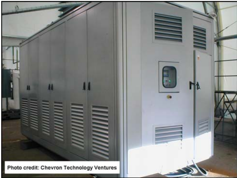
Figure C-2 Primary reformer at Chevron – AC Transit Hydrogen Energy Station (75 kg/day)
