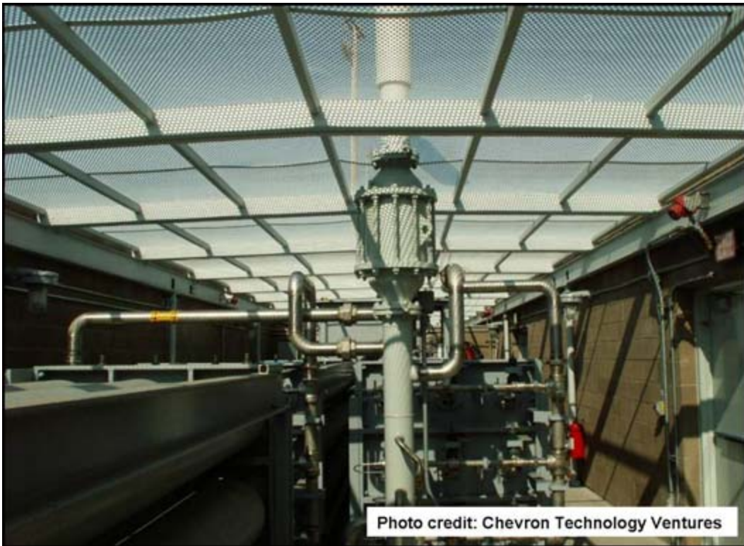
Figure C-3. Cascade hydrogen storage vessels at AC Transit station
