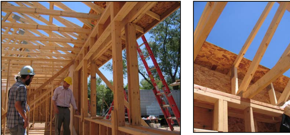
Figure 4. Photograph showing stud wall and raised heel truss construction
