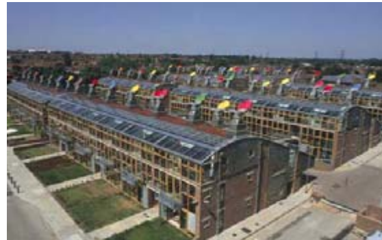
BedZED building in progress. © Arup/Graham Gaunt
